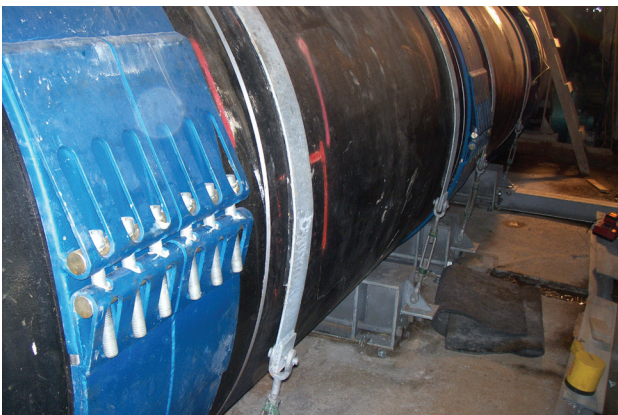
STRAUB-FLEX used as a compensator on unstable ground
