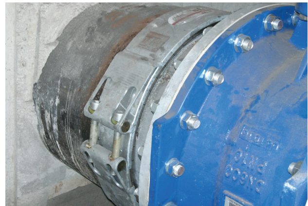
Compensation of diameter differences when installing controls and instruments
