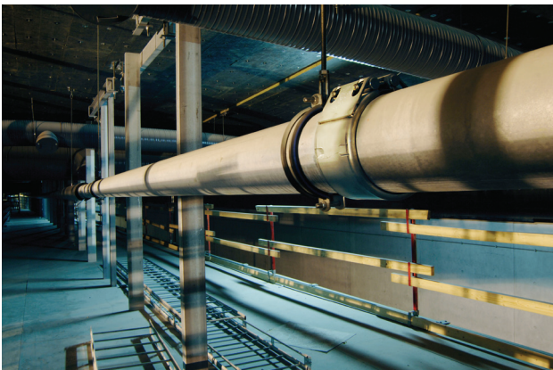
STRAUB-METAL-GRIP as a high-quality pipe joint in a tunnel area; shock proofed up to 200 g
