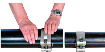
Slide the connectors over both pipes.
